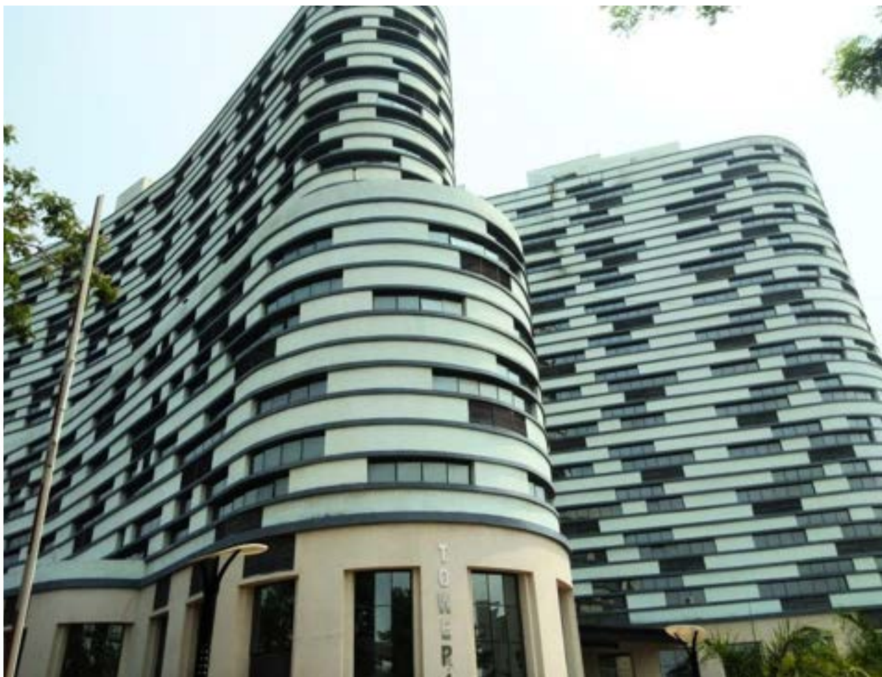
The office space for Bhubaneswar Zonal office
